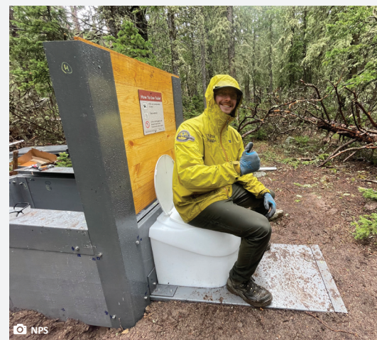
Rocky's wilderness crews installed five new toilets in 2025.
